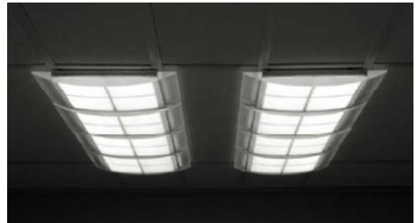
UDC/Armstrong luminaire – 51 lm/W Snaps into TechZone ceiling
